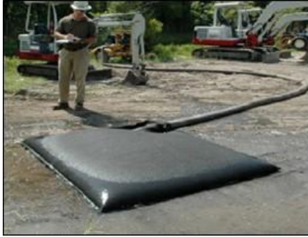
Plate 4-3 Silt Bag with water being pumped through
