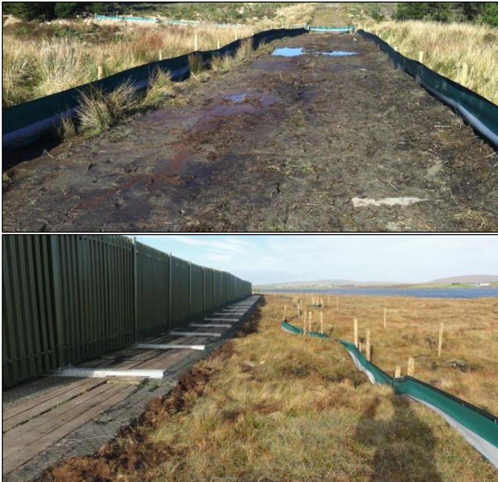
Plate 4-6 Silt Fence Details
