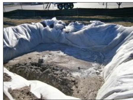
Plate 4-2 Concrete washout area
