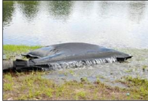
Plate 4-4 Silt bag under inspection
