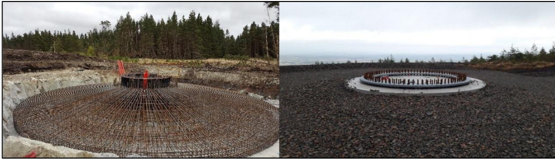
Plate 4-1 Turbine 'Anchor Cage' and finished turbine base
