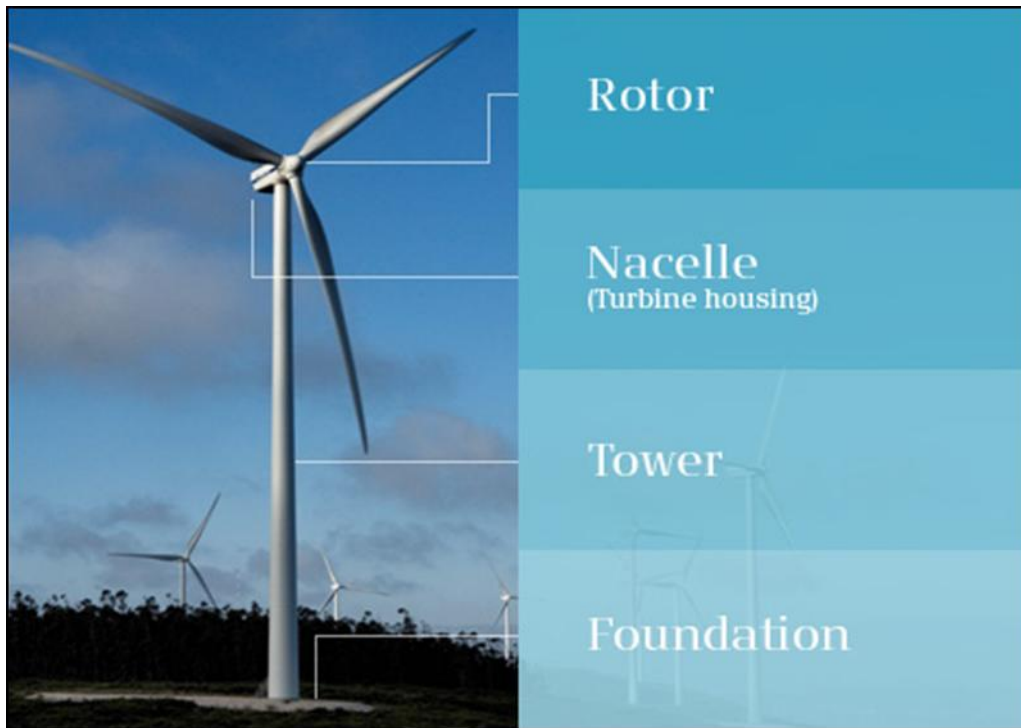
Figure 4-2: Wind Turbine Components
