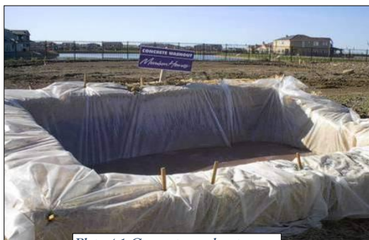
Plate 4-1 Concrete washout area
