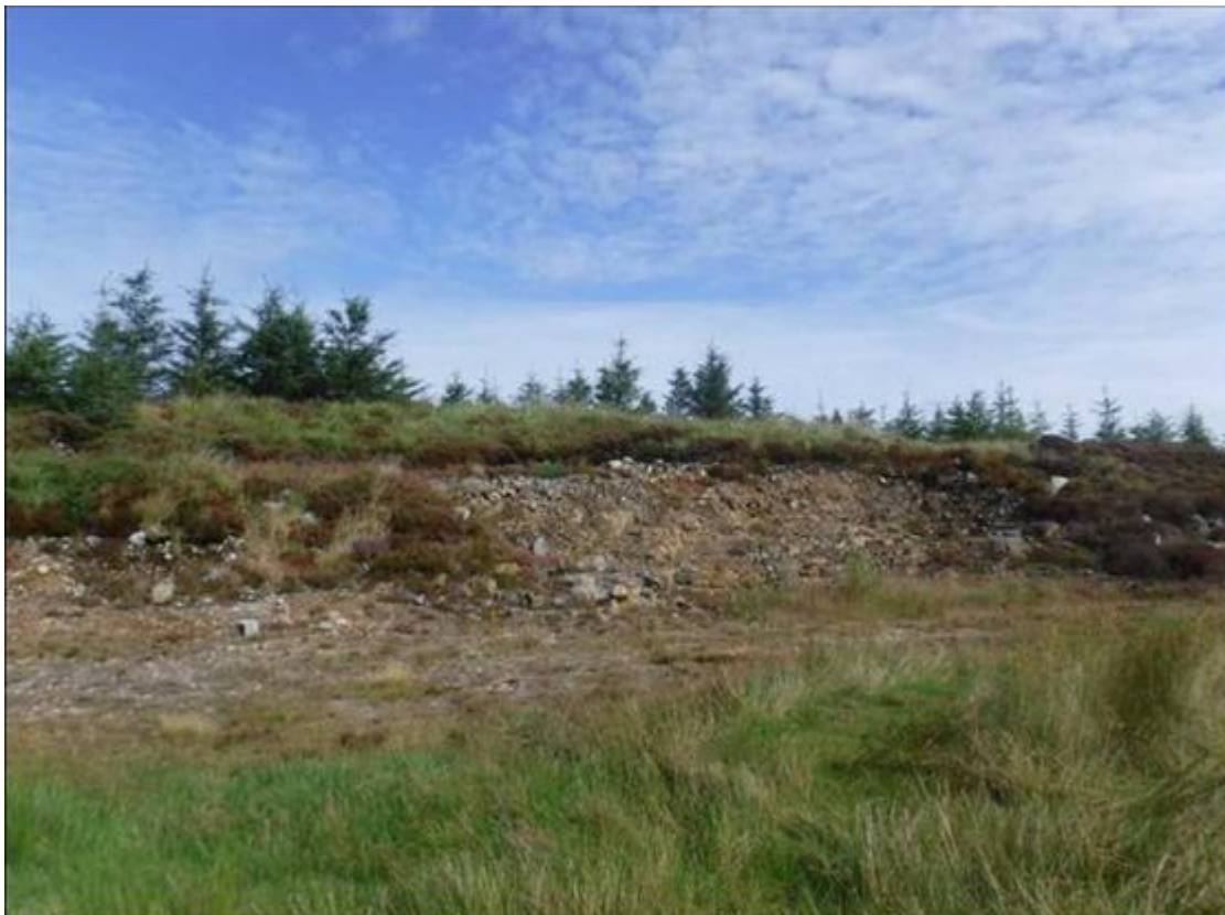
Plate 8-1: Bedrock Exposures at Proposed Borrow Pit 2 (Photograph taken from south of BP location)
