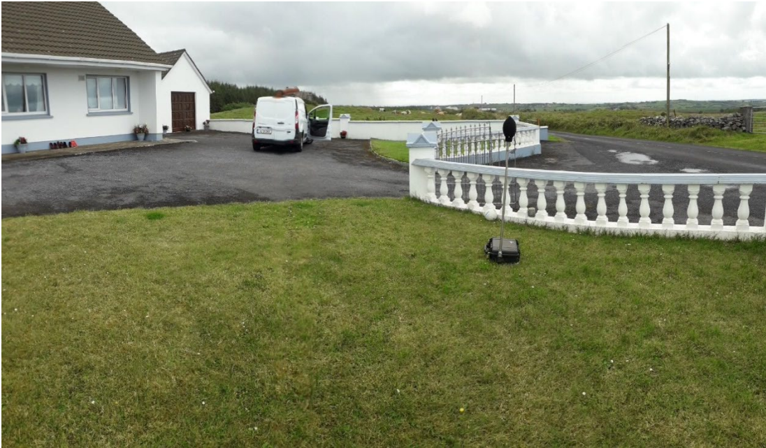
Appendix Figure B-6. Location D Installation
