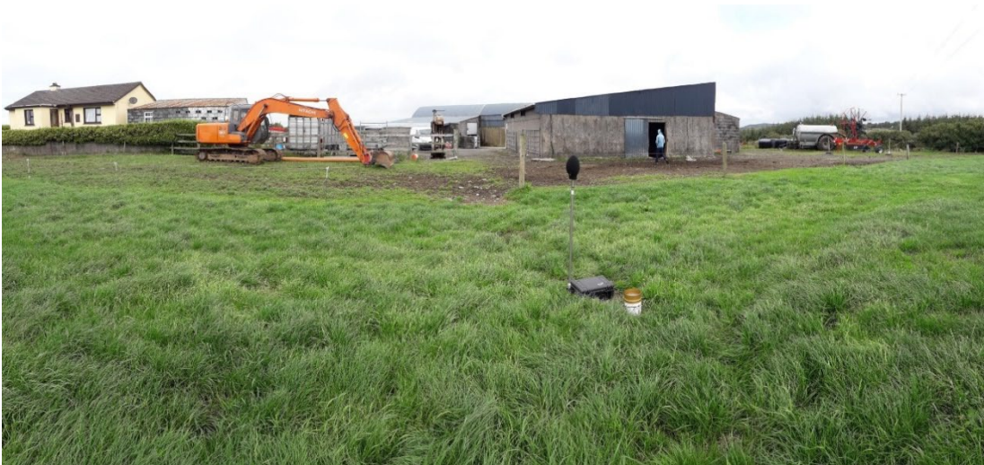
Appendix Figure B-7. Location E Installation
