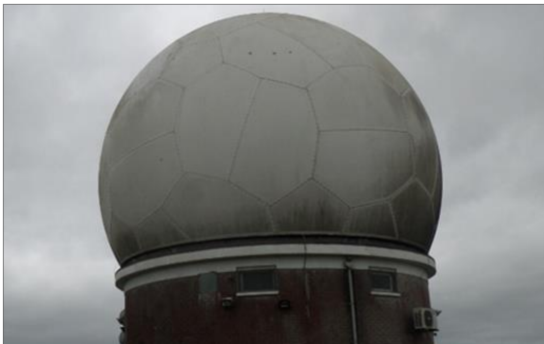
Figure 15. Woodcock Hill Airport - Secondary Surveillance Radar (SSR)
