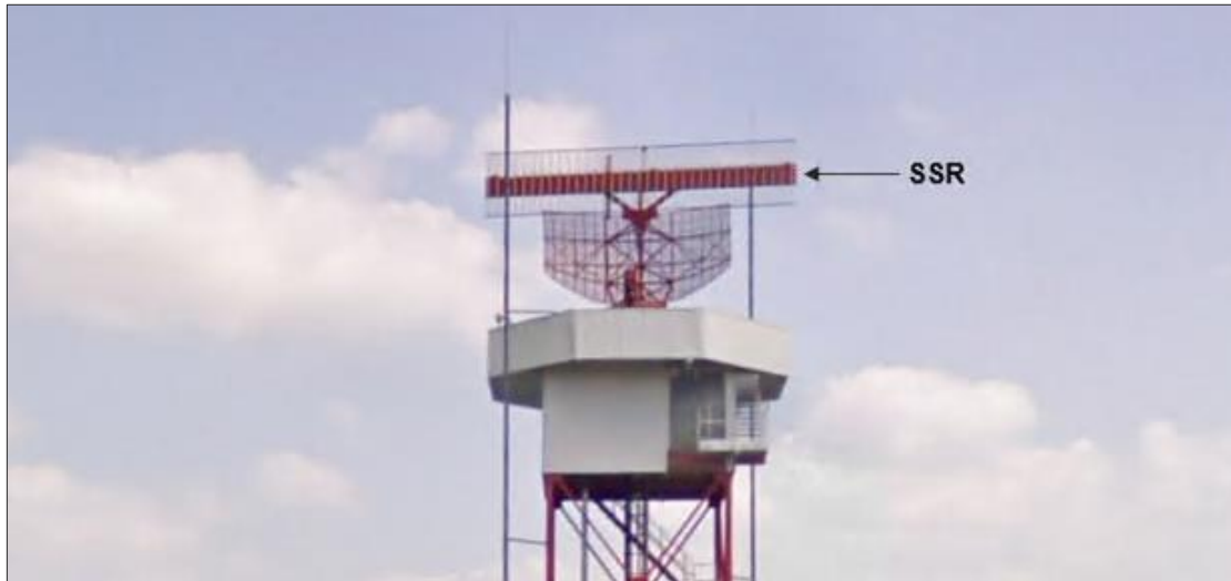
Figure 14. Shannon Airport - Secondary Surveillance Radar (SSR)
