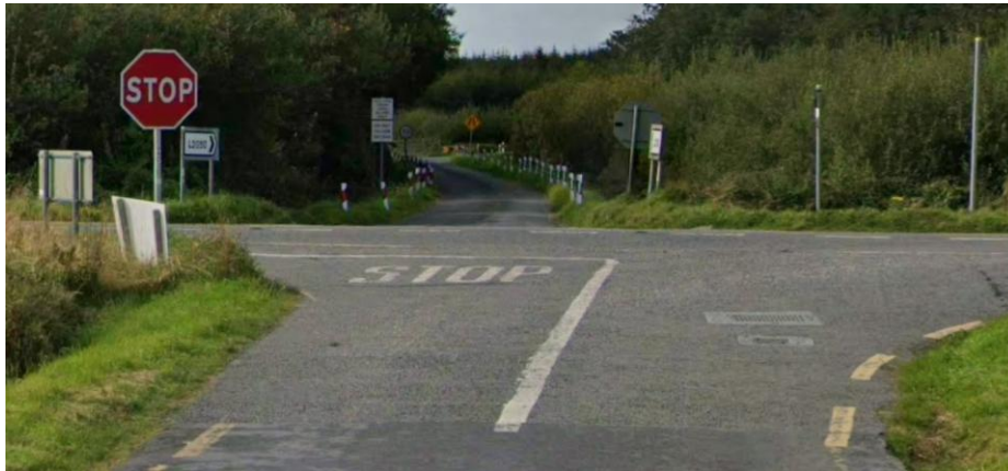
Figure 15 National Road (N-68)
