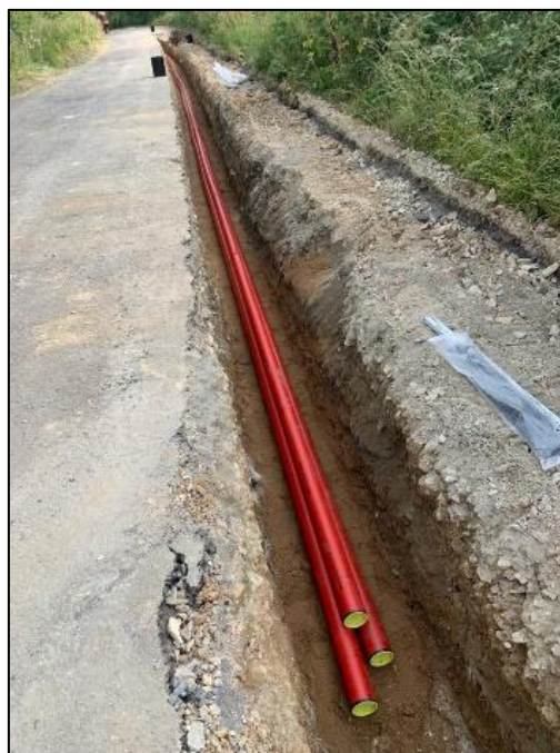
Figure 3 Typical 110kV Underground Duct Installation
