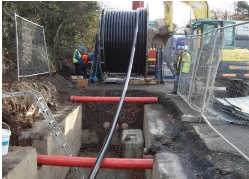
Figure 9 Typical Cable Pulling Drum Set Up
