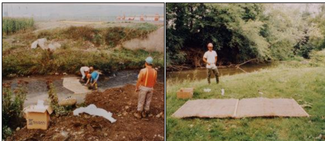
Plate 2-3 Typical Sedimat Details (Source: https://www.hy-tex.co.uk/ )
