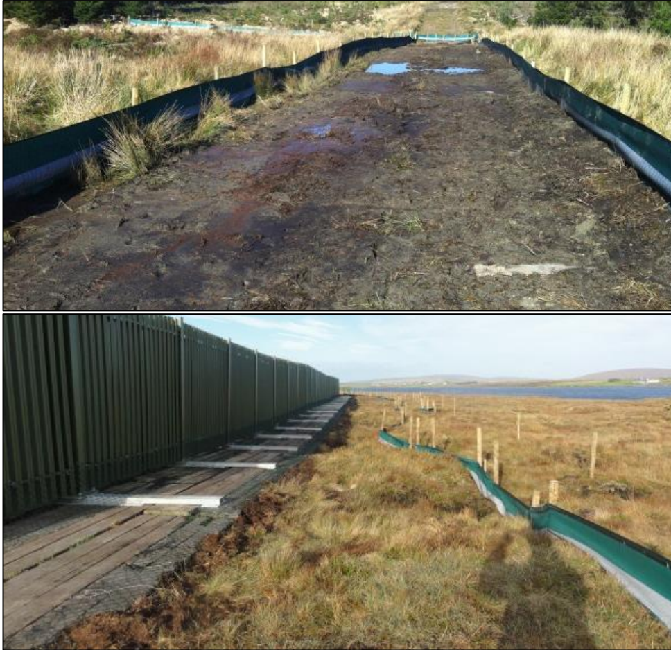
Plate 2-4 Typical Silt Fence Details
