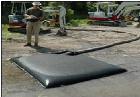
Plate 2-1 Silt Bag under inspection
