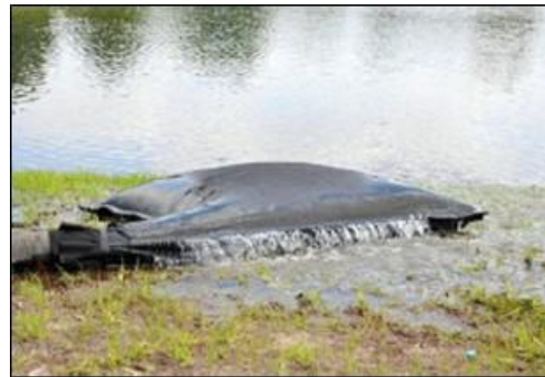
Plate 2-2 Silt Bag with water being pumped through
