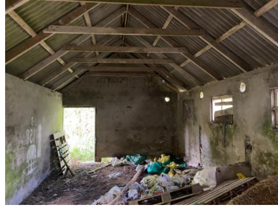
Plate 4-11 Internal condition of Structure No. 1
