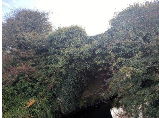
Plate 4-8 Stone single-arched bridge at WC20 showing stonework partially obscured by vegetation, with a small number of exposed crevices above the waterline, assessed as offering Low bat roosting potential.
