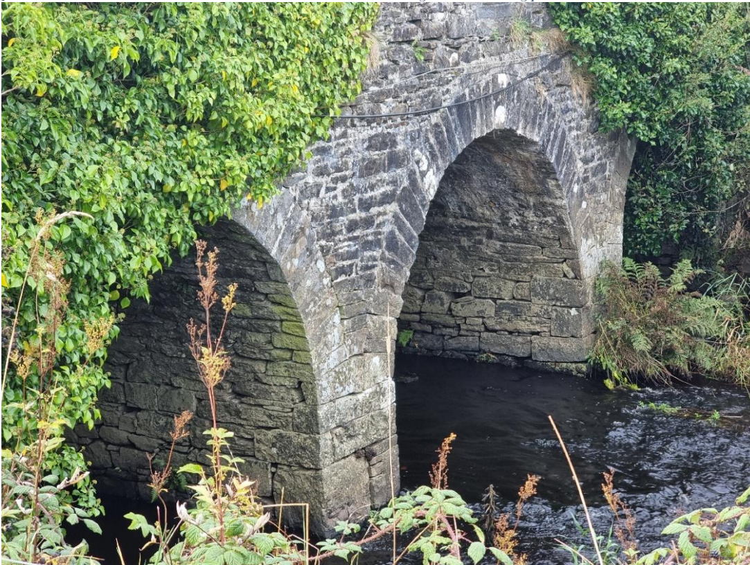
Plate 4-9 Stone triple-arched bridge at WC14 showing recessed mortar joints and crevices above the waterline, assessed as offering Moderate bat roosting potential.
