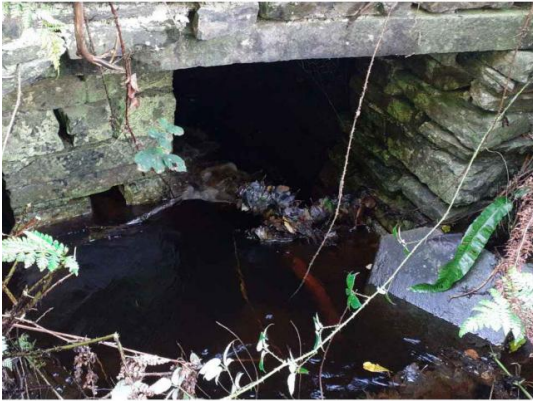
Plate 4-5 Double stone clapper at WC7 showing exposed stonework and localised gaps between stones above the waterline, assessed as offering Low bat roosting potential.
