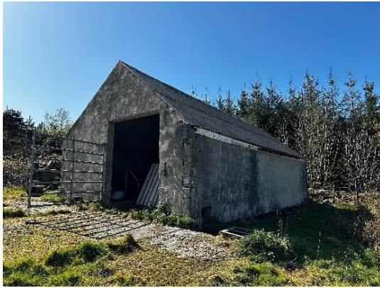
Plate 4-14 Northeast aspect of Farm Shed A (Structure No. 2)
