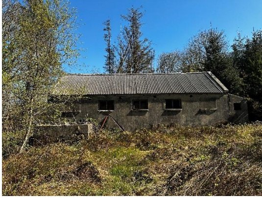
Plate 4-10 West aspect of Farm Building (Structure No. 1)
