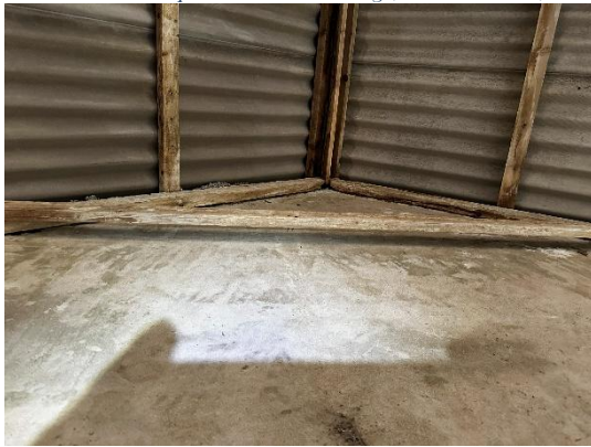
Plate 4-12 Potential roosting spaces within Structure No. 1 between end rafters and walls
