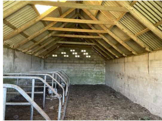
Plate 4-15 Interior of Farm Shed A showing roof structure
