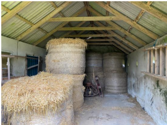
Plate 4-20 Interior of Farm Shed B
