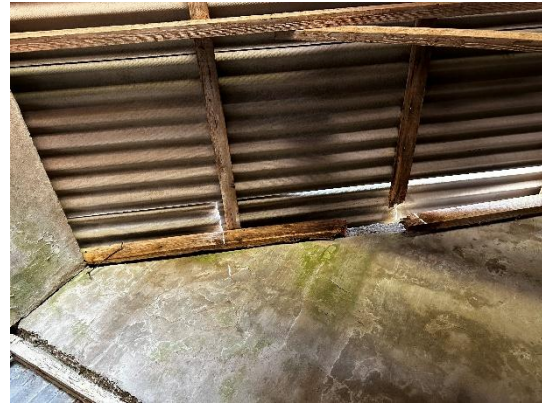
Plate 4-19 Potential roosting spaces within Structure No. 3 between end rafters and walls
