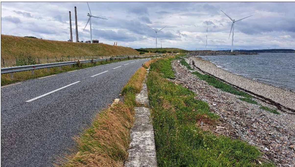
Plate 3.23 Representative image of site D15, July 2024 (culverted underground)
