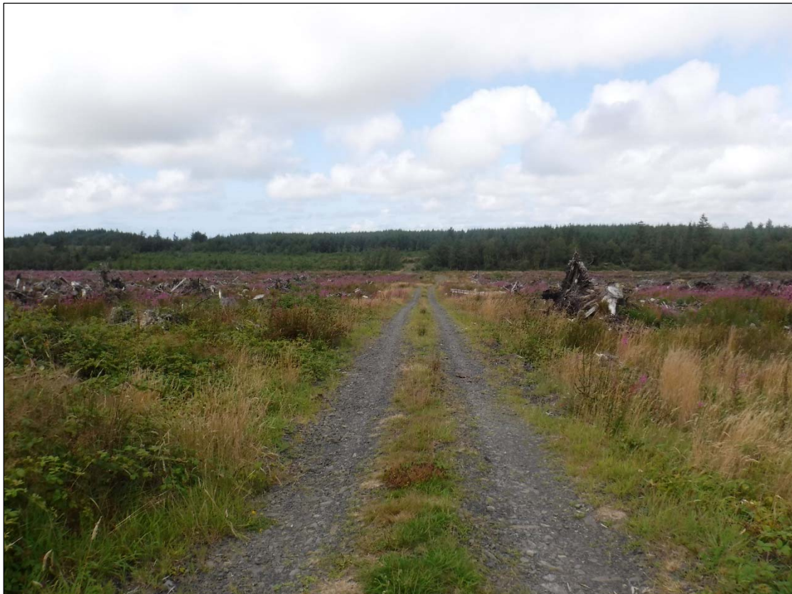
Photo 4: Looking North along existing access road at T07
